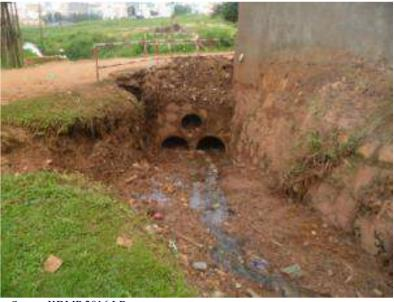
Source KDMP 2016 LR Figure 14.3.7 Deposit of Sediment in Drainage Channel
